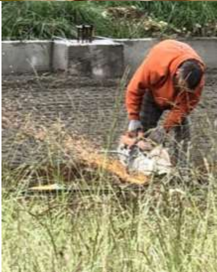
It takes a whole lot of rebar to prepare the foundation!
